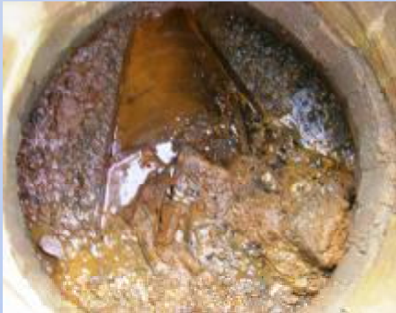
Main Post – MH 9E (Riverside Avenue) Estimated 2 gpm (3,000 gpd) from caps of both pipes.
