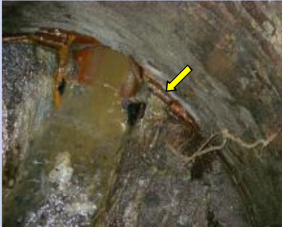
Charles Wood – MH 44B (Hemphill Road) Arrow points to estimated 2 gpm (3,000 gpd) wall leak to right of effluent pipe. Minor root intrusion from wall / bench junction.
